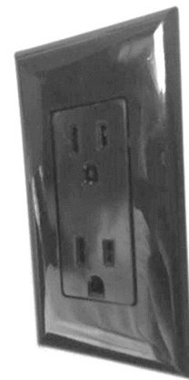
Figure 6-6: 120 VAC Receptacle
