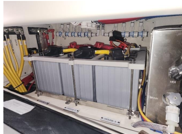
Hot & Cold Water Manifold
