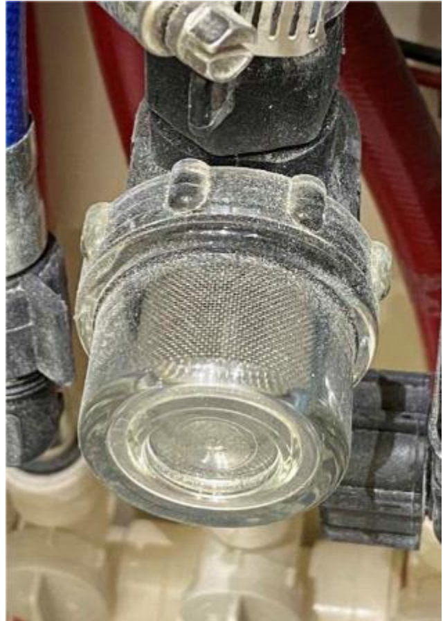
Fresh Water Pump Strainer
