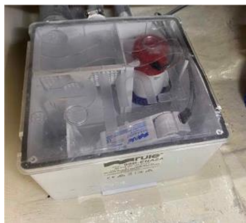
Shower Sump System including Pump
