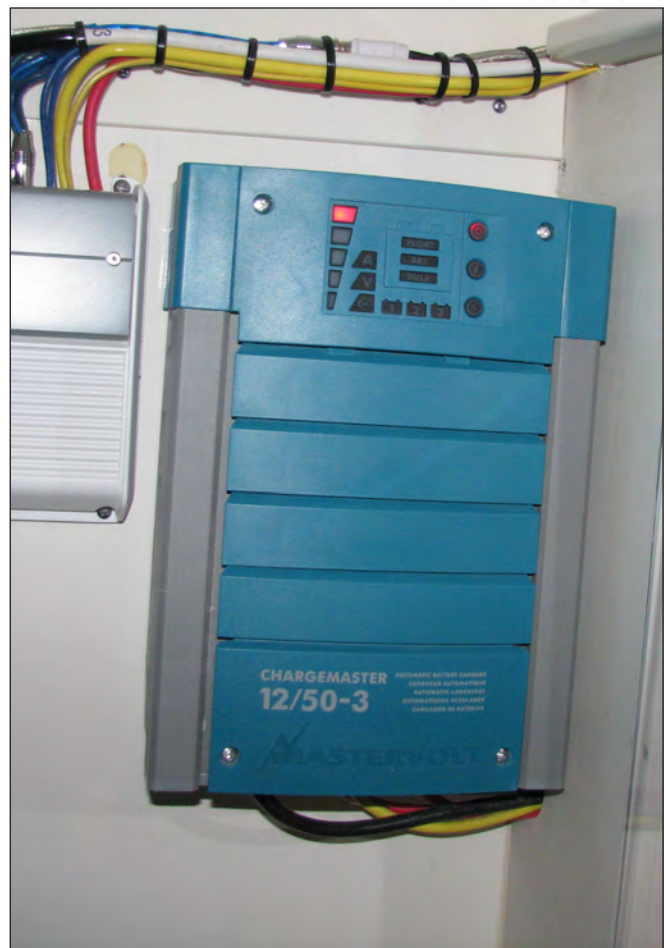
Typical Battery Charger
