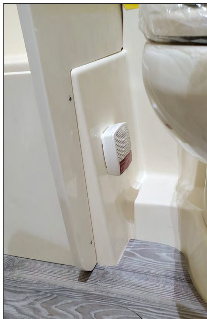
Typical Carbon Monoxide Detector & Alarm
