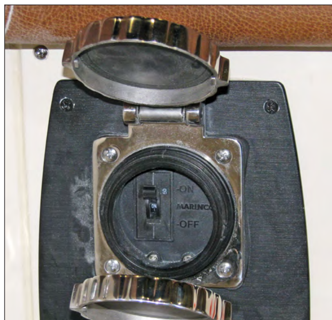
Shore Power Inlet Circuit Breaker
