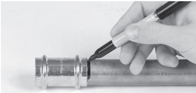
Figure 8 – Marking the Tubing After Fully Inserting Tube
