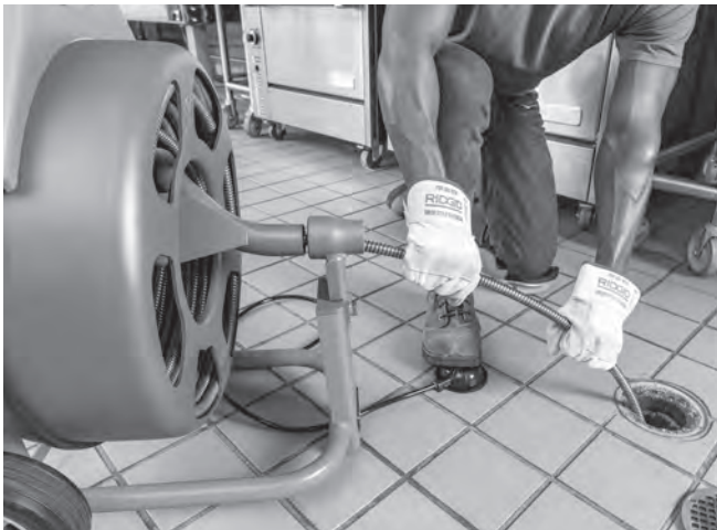
Figure 13 – Feeding of the Cable
