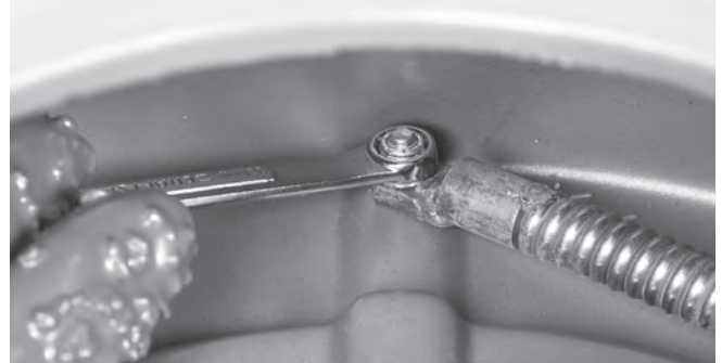
Figure 30 – Pigtail Anchor Bolt
