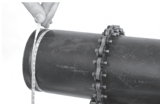
Figure 18 – Checking Groove Diameter with a Diameter Tape
