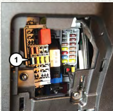
Interior Fuse Panel Power Outlet Fuse
