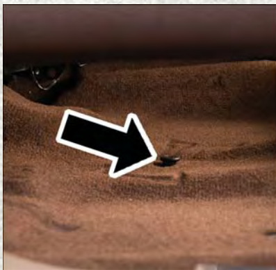
Floor Fastener Location
