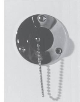
Washdown Hose Connector (Typical)
