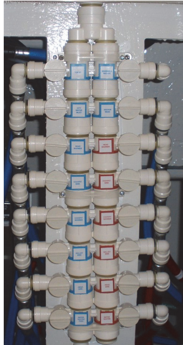
Water System Manifold (Typical)
