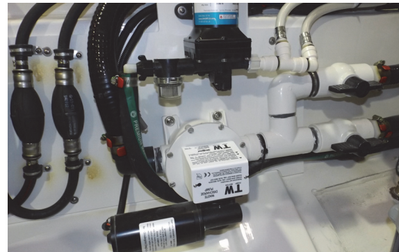
Fishbox Drain Manifold
