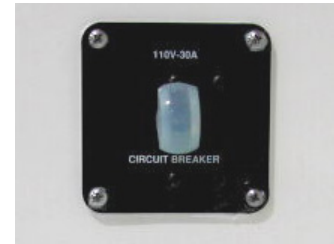
Shore Power Breaker
