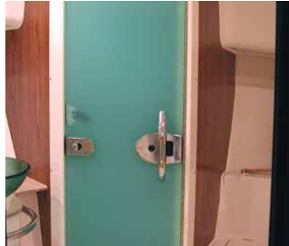
Shower and Linen Lock Door and Latches
