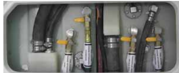
Fuel Tank Valves
