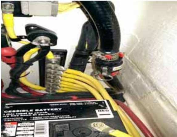
Rear Storage Drain
