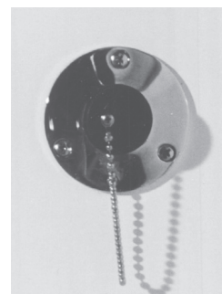
Washdown Hose Connector (typical)
