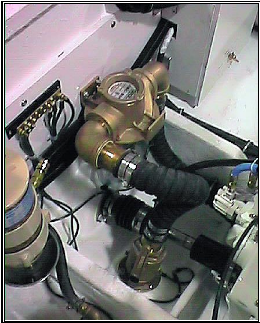
Figure 6-6: Engine Raw Water Intake
