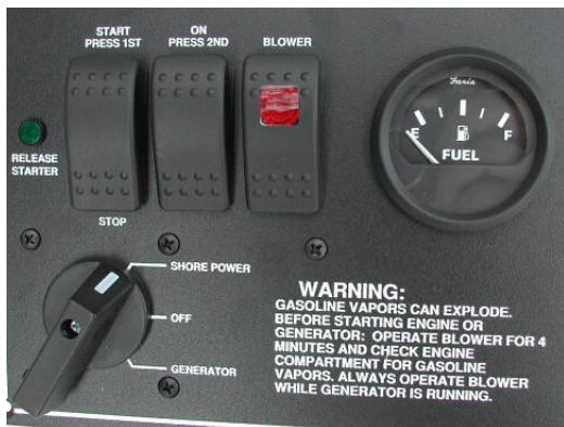
Gasoline Generator Panel
