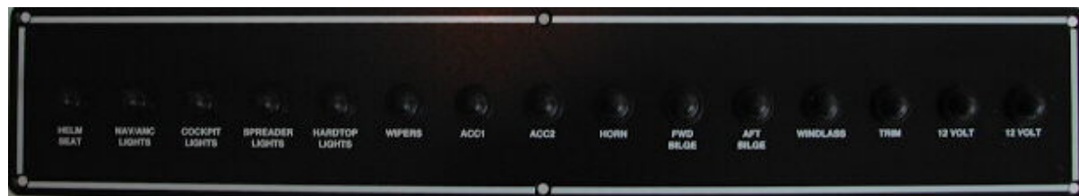
Helm Breaker Panel
