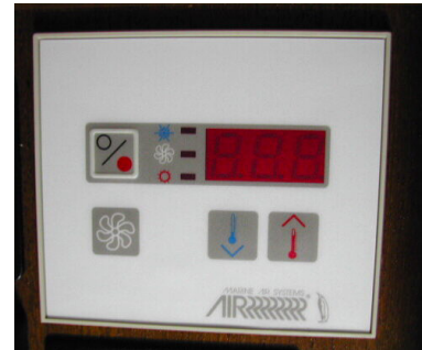
Air Conditioning Control Panel
