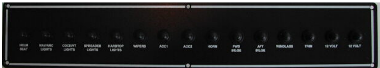
Helm Breaker Panel
