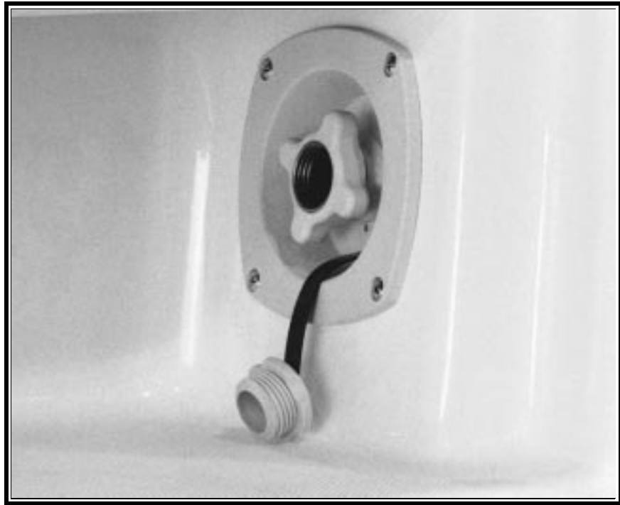
Figure 1-16: Dockside Water Inlet
