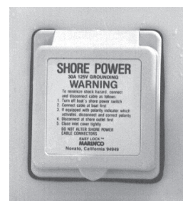
Shore Power Inlet
