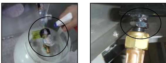
Gas Connection Leak Check
