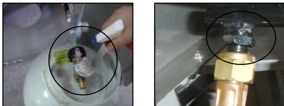
Gas Connection Leak Check
