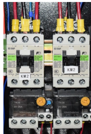
Figure 5-3: Vacuum Pump Contactor(s) with electrical wires and ground attached
