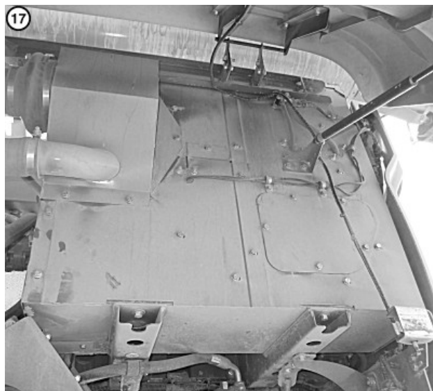
(17) — Areas around and under Exhaust Aftertreatment Enclosure (if equipped)
