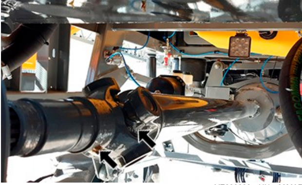
YE000683—UN—30MAR23 Driveshaft End and Splined Rod (2 greasing points)— Machines Equipped with Front Engine
