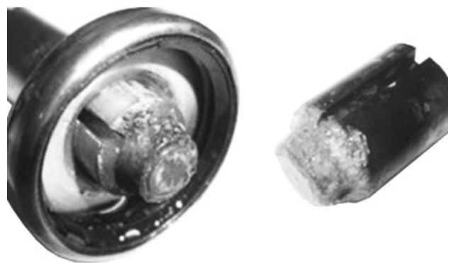
Heavy Corrosion and Pitting
