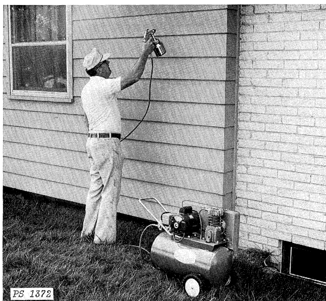
Using the Compressor, Spray-Painting
