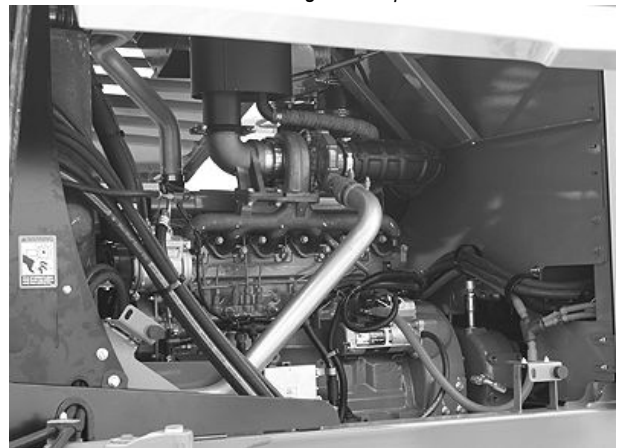
Right Side Engine Compartment
