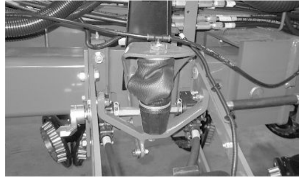
Improperly Rolled Air Spring
