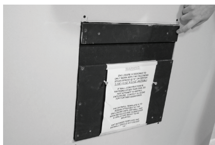
Figure 25 Install surrounding wallboard flush against wallboard template.
