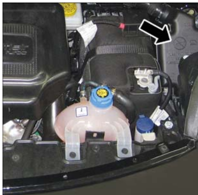
Front Distribution Unit
