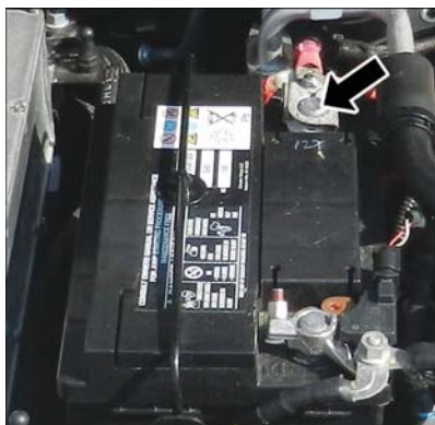
Positive Battery Post
