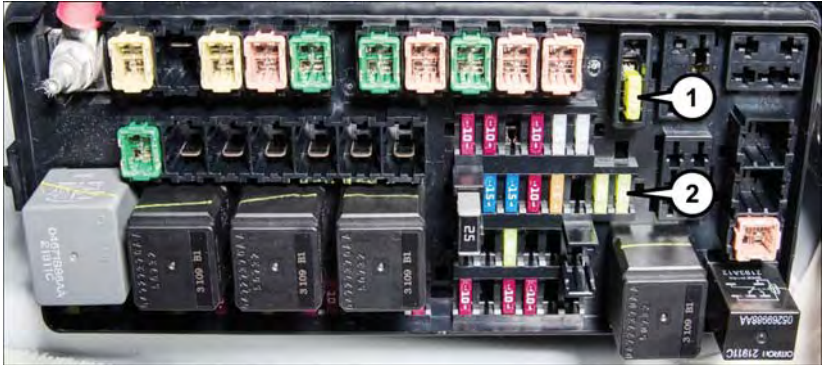
Power Outlet Fuses
