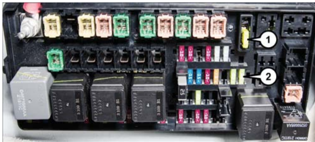
Power Outlet Fuses
