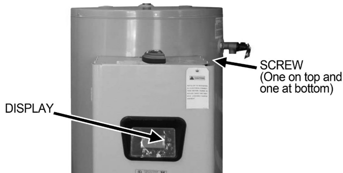
Figure 26. Loosening the Screws to the Door of the Unit
