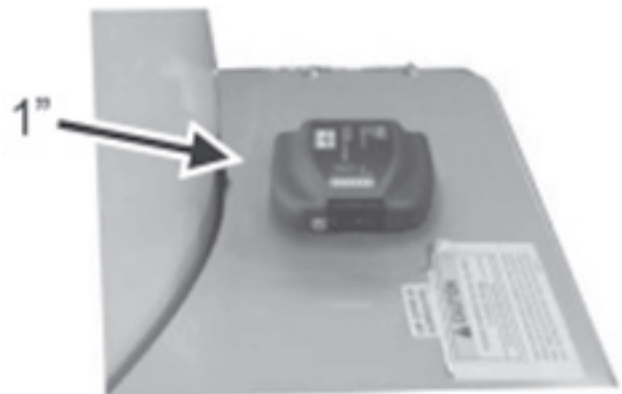
Figure 18. ICC Location Relative to Water Heater Jacket
