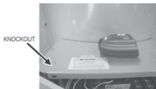
Figure 20. Location of Communications Wiring Knockout
